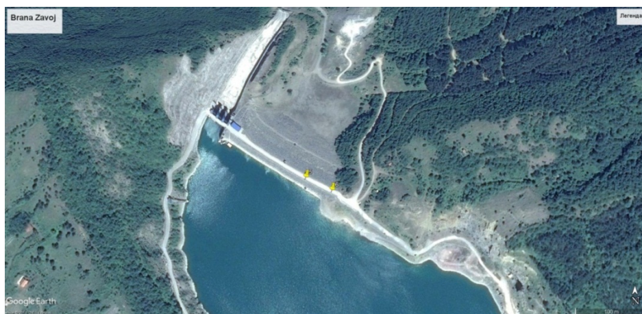
Figure 1. Large dam “Zavoj” with position of benchmarks
