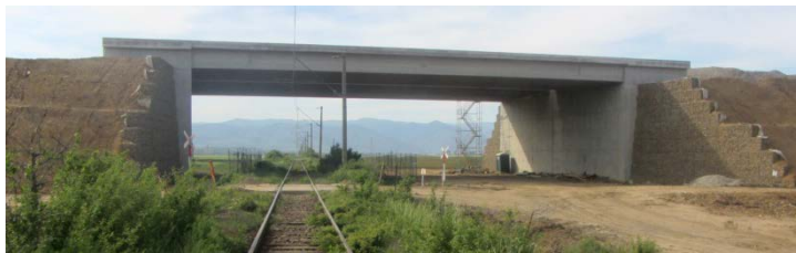
Figure 11 One spanned motorway bridge, deck with prefabricated prestressed girders
