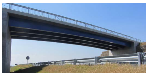
Figure 9 Motorway overpass, Composite integral bridge L = 39 m
