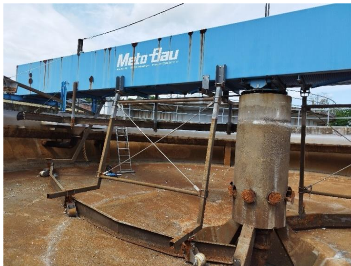
Figure 3: Wear of the tank's bottom plate along the wheels
