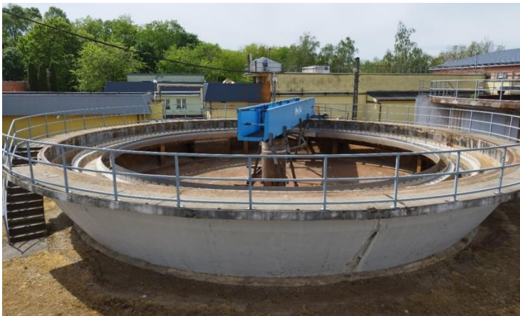
Figure 1: The number three primary settling tank
