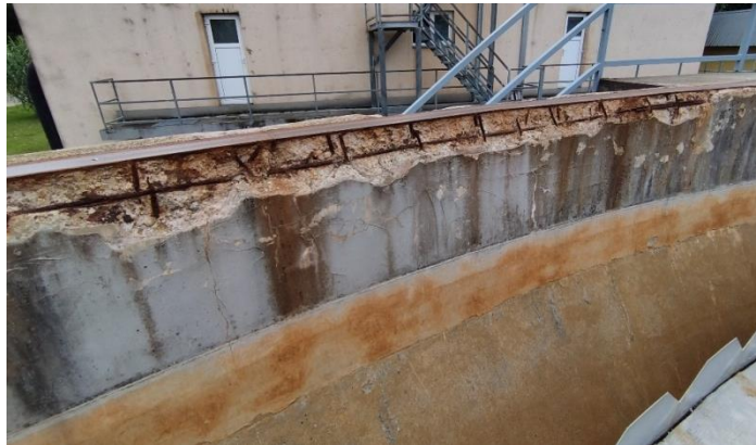
Figure 2: The missing concrete cover from the inner part of the tank edge
