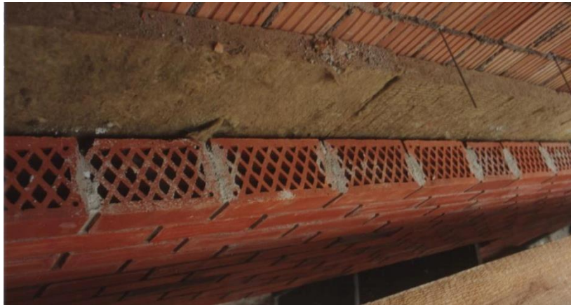
Figure 2: Paving brickwork during construction 2
