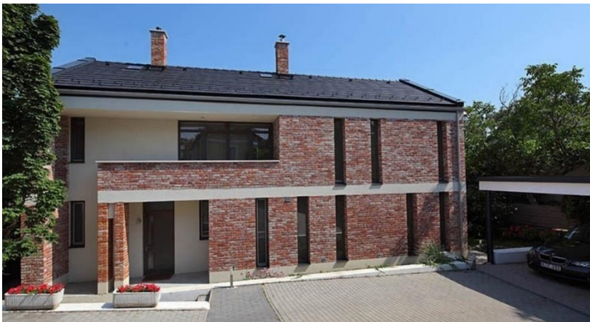
Figure 3: ventilated facade brickwork, the completed building 3
