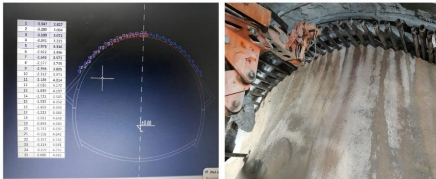
Figure 2: Tube layout foreseen by the project
