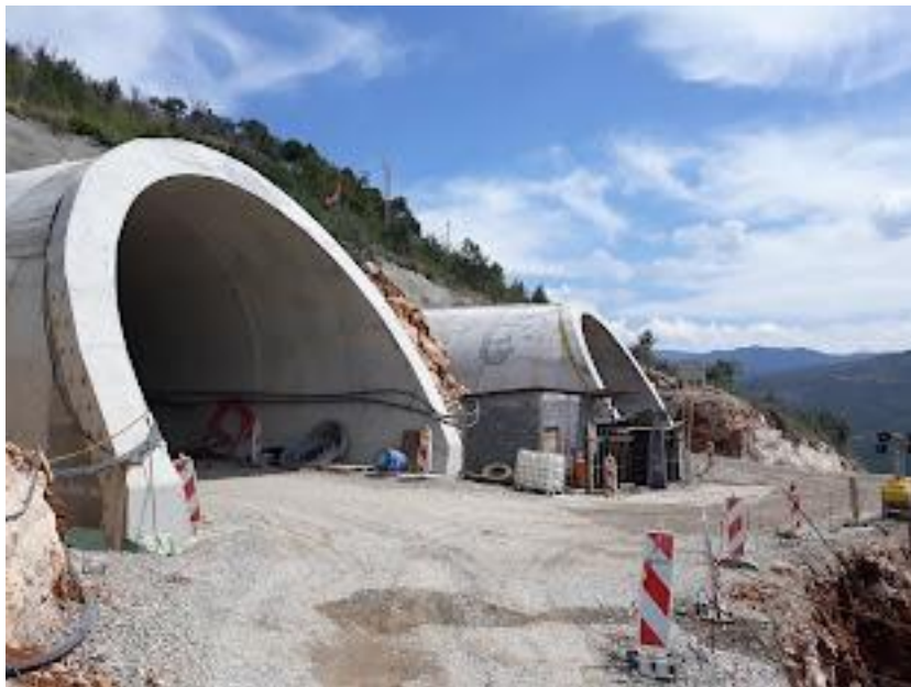
Figure 1: Entry portals of the tunnel
