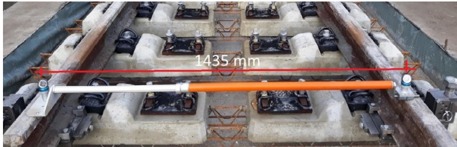
Figure 3: Positioning of rails
