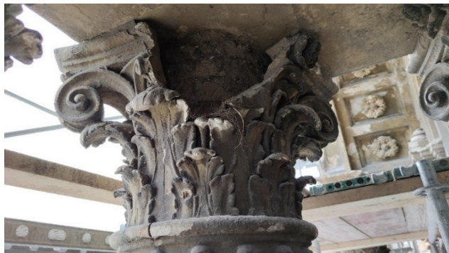
Figure 5. Column head damage
