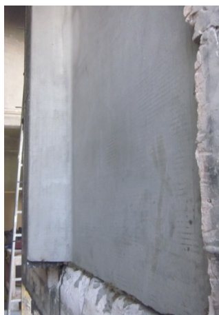
Figure 5. The 2 nd test - exposed side
