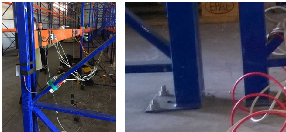
Figure 3. Tested steel rack: beam-to-column connection (left) and column-to-floor connection (right)
