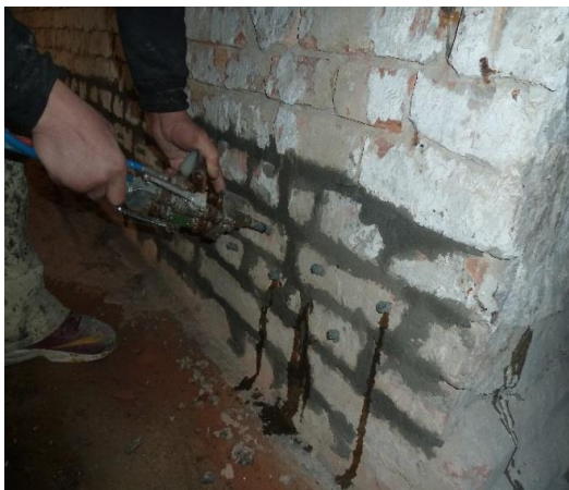
Figure 12. Brick basement wall with MC Bauchemie injection work
