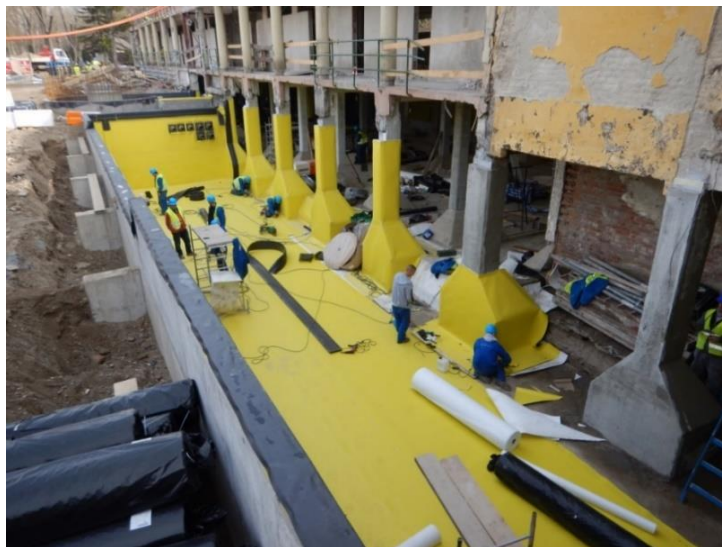
Figure 11. Hydro-isolation work of north-wing of Palatinus bath
