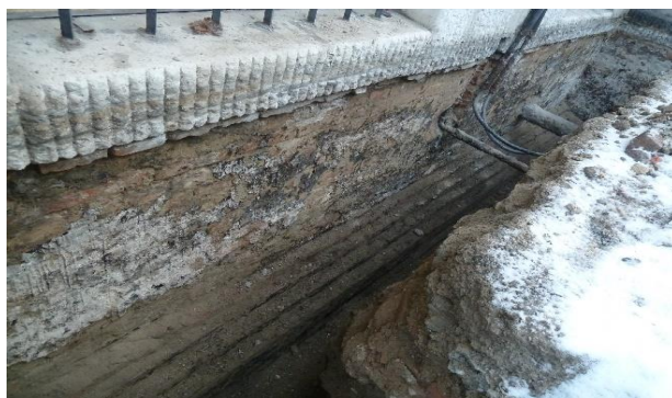
Figure 13. The street side water insulation
