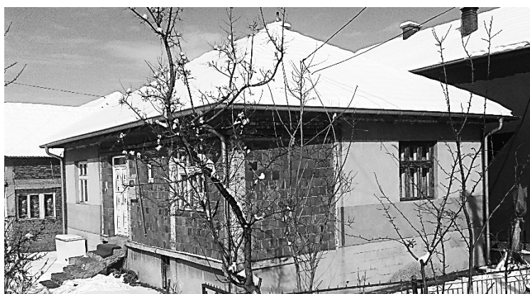
Figure 15. Rehabilitated house with a new roof structure
