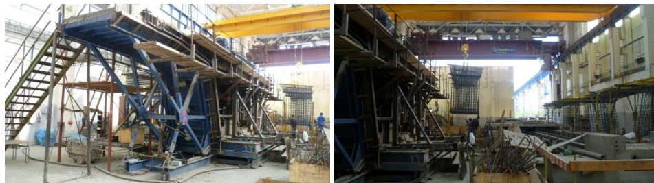
Figure 2. Segments casting in in adjustable molds
