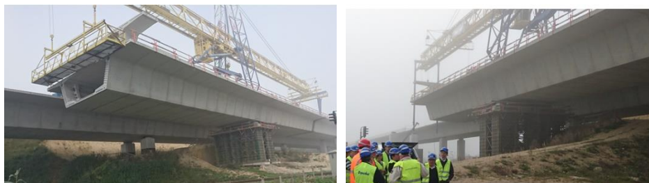
Figure 3. Self-launching gantry with centre leg on pier transporting a segment
