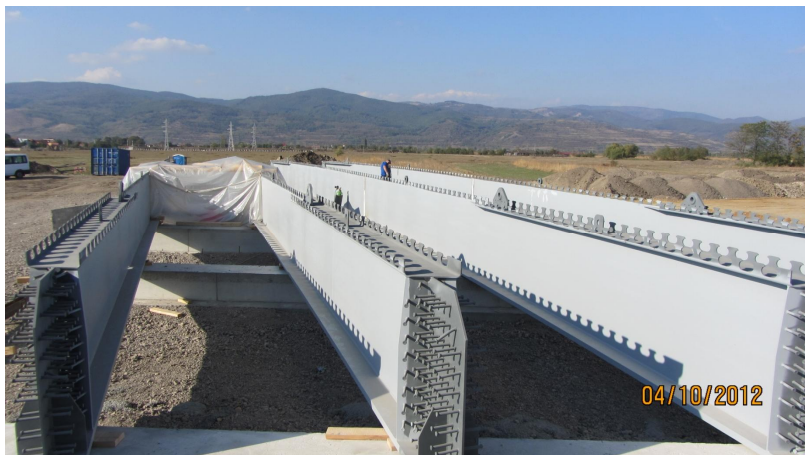
Fig. 8 Steel girders on the site, ready for erection.
