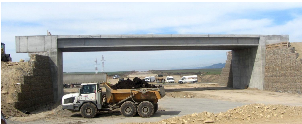
Fig 6 Overpass on the national road – site photo
